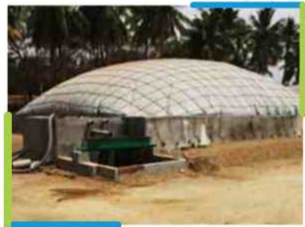
Conventional Bio-gas Plant 1 TPD – 100 TPD
